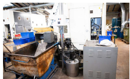
Picture of our high-end external machine connection for ensuring efficient exchange and filtering.
